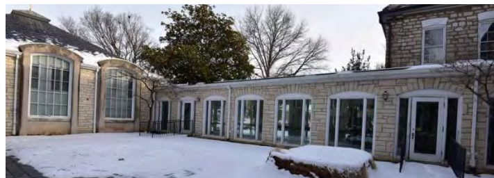
Figure 23: Resource 1, Block G, north and west elevations. Source: Brad Finch, F-Stop Photography, March 2015.
