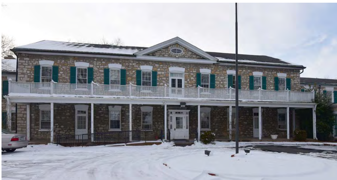
Figure 7: Resource 1, Block A, east elevation. Source: Brad Finch, F-Stop Photography, March 2015.
