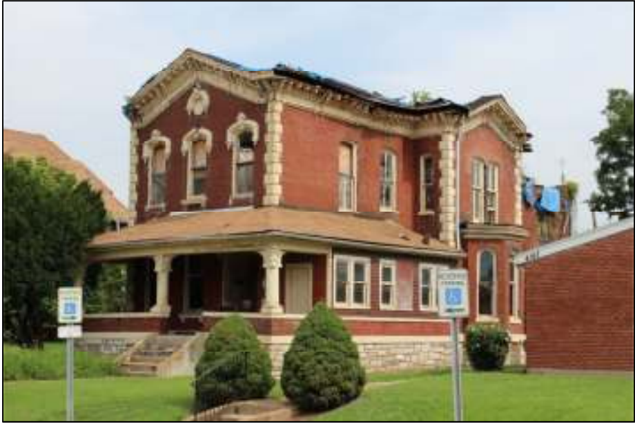
4171 WEST BELLE – EAST FAÇADE
