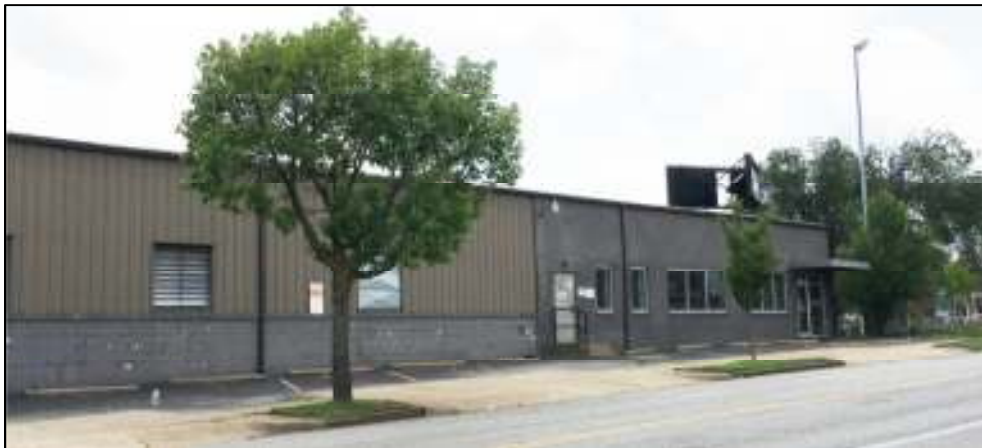
INDUSTRIAL BUILDING AT 1302 RUSSELL
