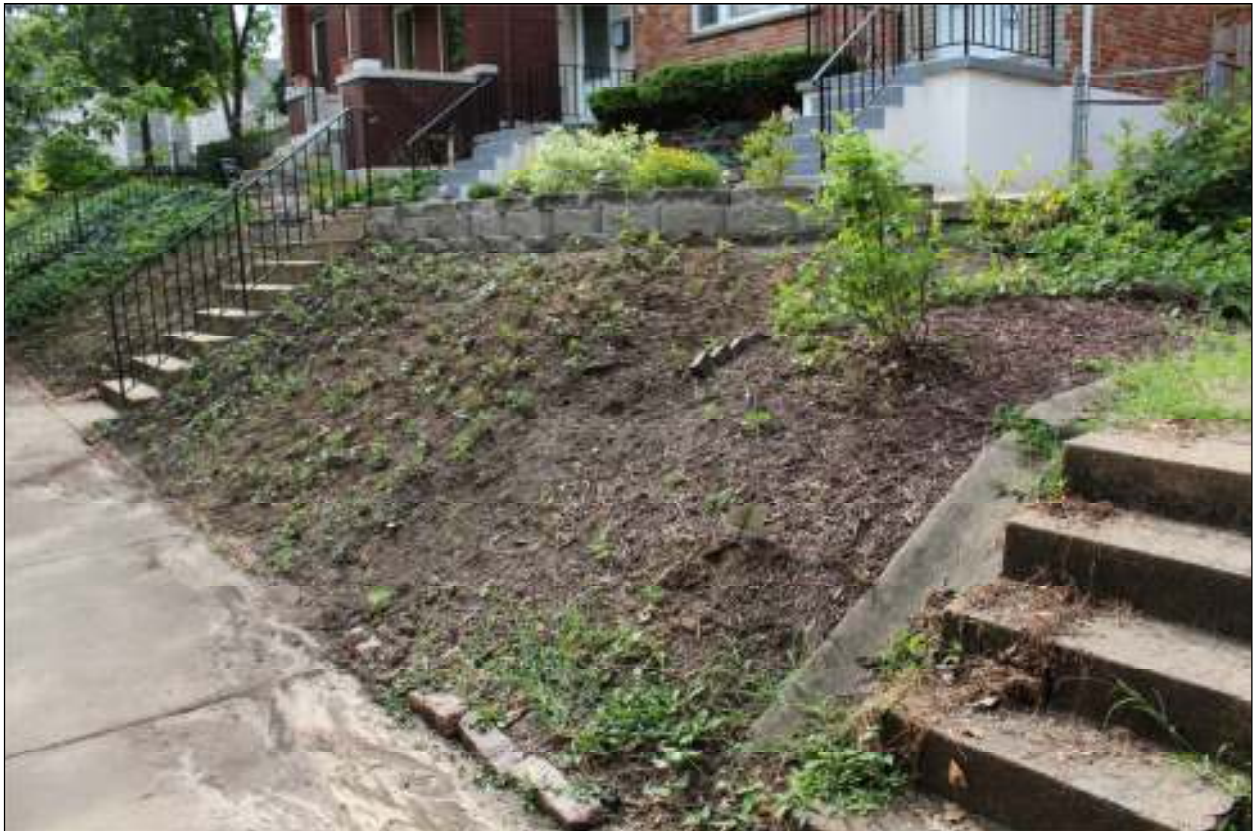
SIDE VIEW OF WALL
