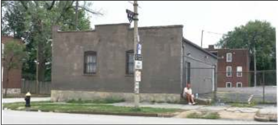
SMALLER BUILDING AT RUSSELL AND S. 13 TH STREET
