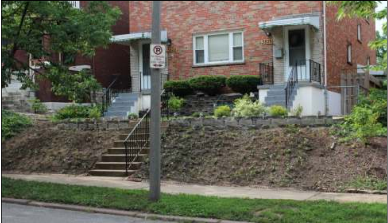
RETAINING WALL INSTALLED WITHOUT A PERMIT
