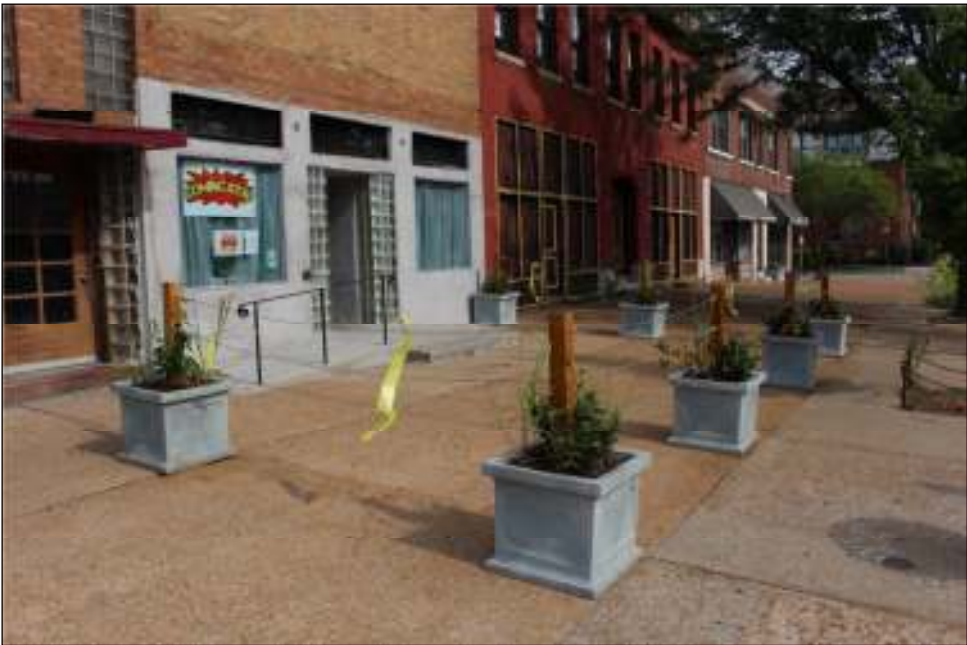
TEMPORARY FENCING INSTALLED IN FRONT OF 2245-47 S. GRAND WITHOUT A PERMIT
