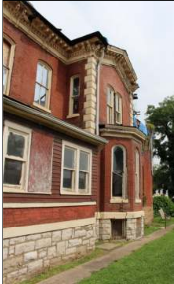
4171 WEST BELLE – EAST FACADE
