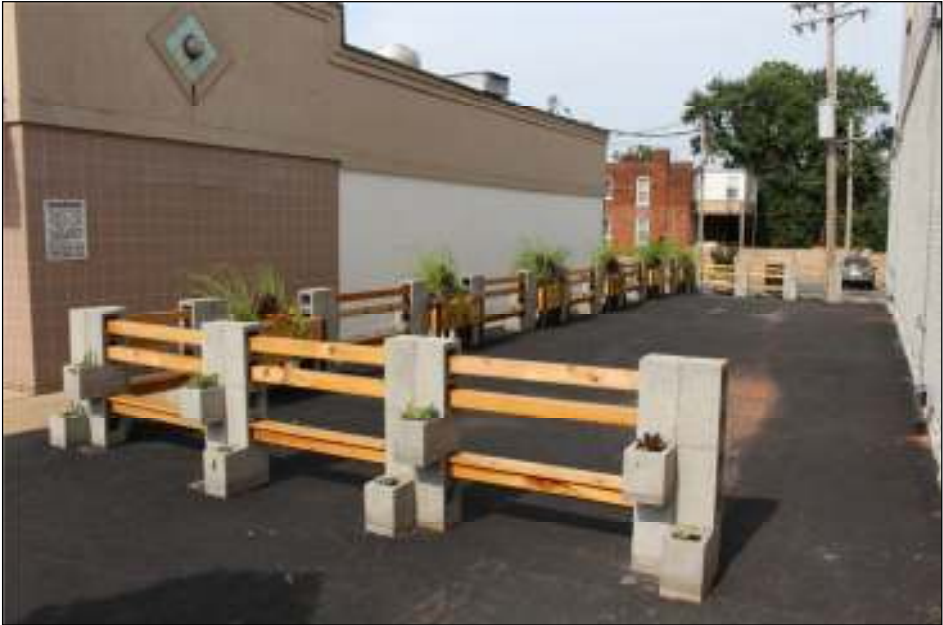
FENCING INSTALLED BETWEEN 2253-55 & 2245-47 S. GRAND BLVD. WITHOUT A PERMIT
