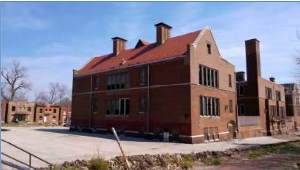
HEMPSTEAD SCHOOL – WEST AND SOUTH FACADES
