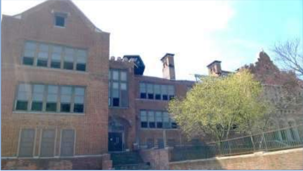
HEMPSTEAD SCHOOL – MAIN FAÇADE DETAIL
