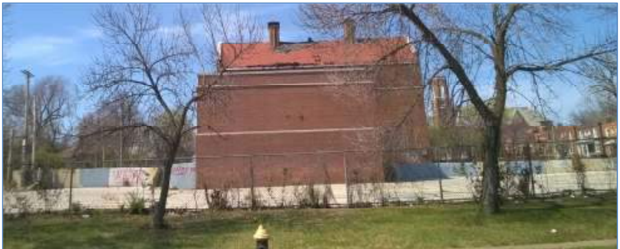
HEMPSTEAD SCHOOL – EAST FACADE
