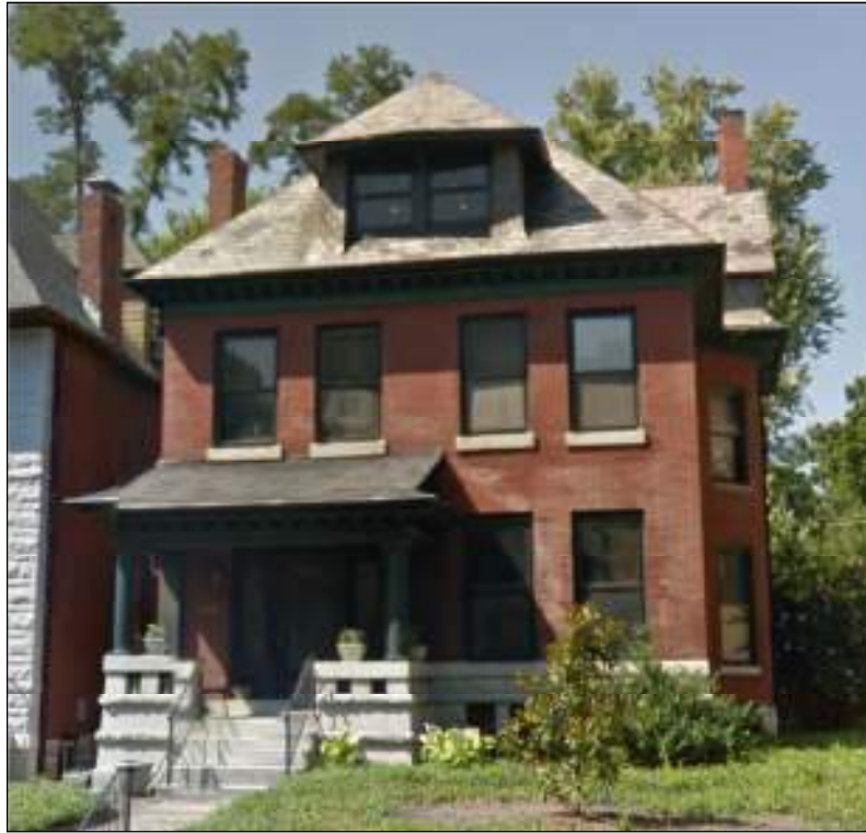
VIEW OF ROOF PRIOR TO REPLACEMENT FROM GOOGLE STREET VIEW JULY 2016
