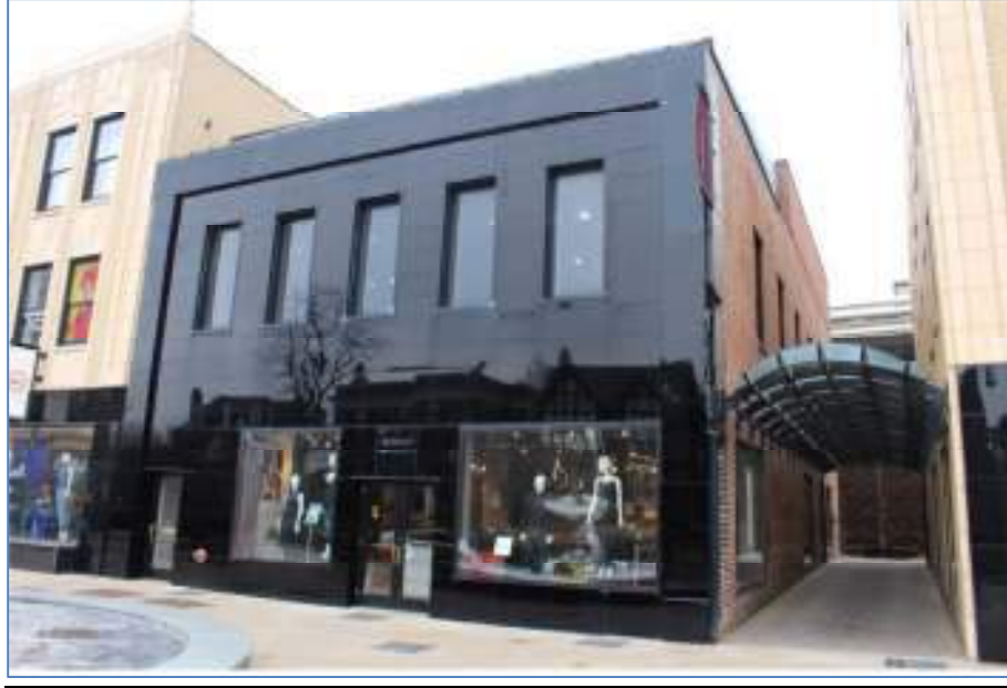
MARYLAND PLAZA FACADE
