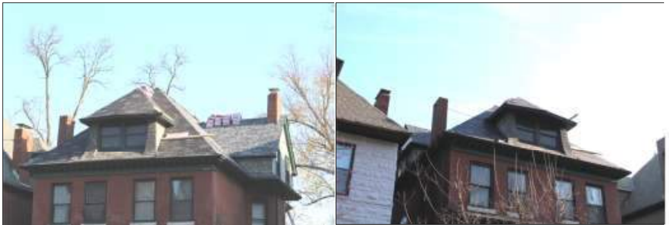
VIEW OF PARTIALLY INSTALLED ROOF
