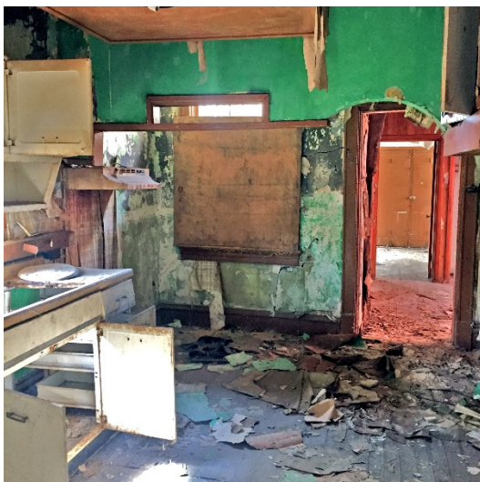
Existing Kitchen Space
