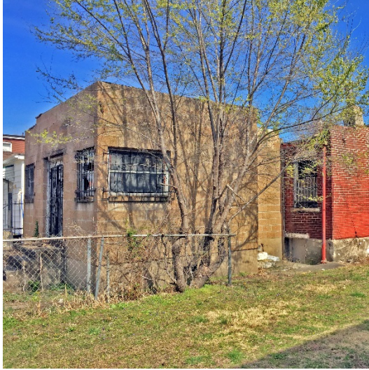
Existing Rear Studio Addition
