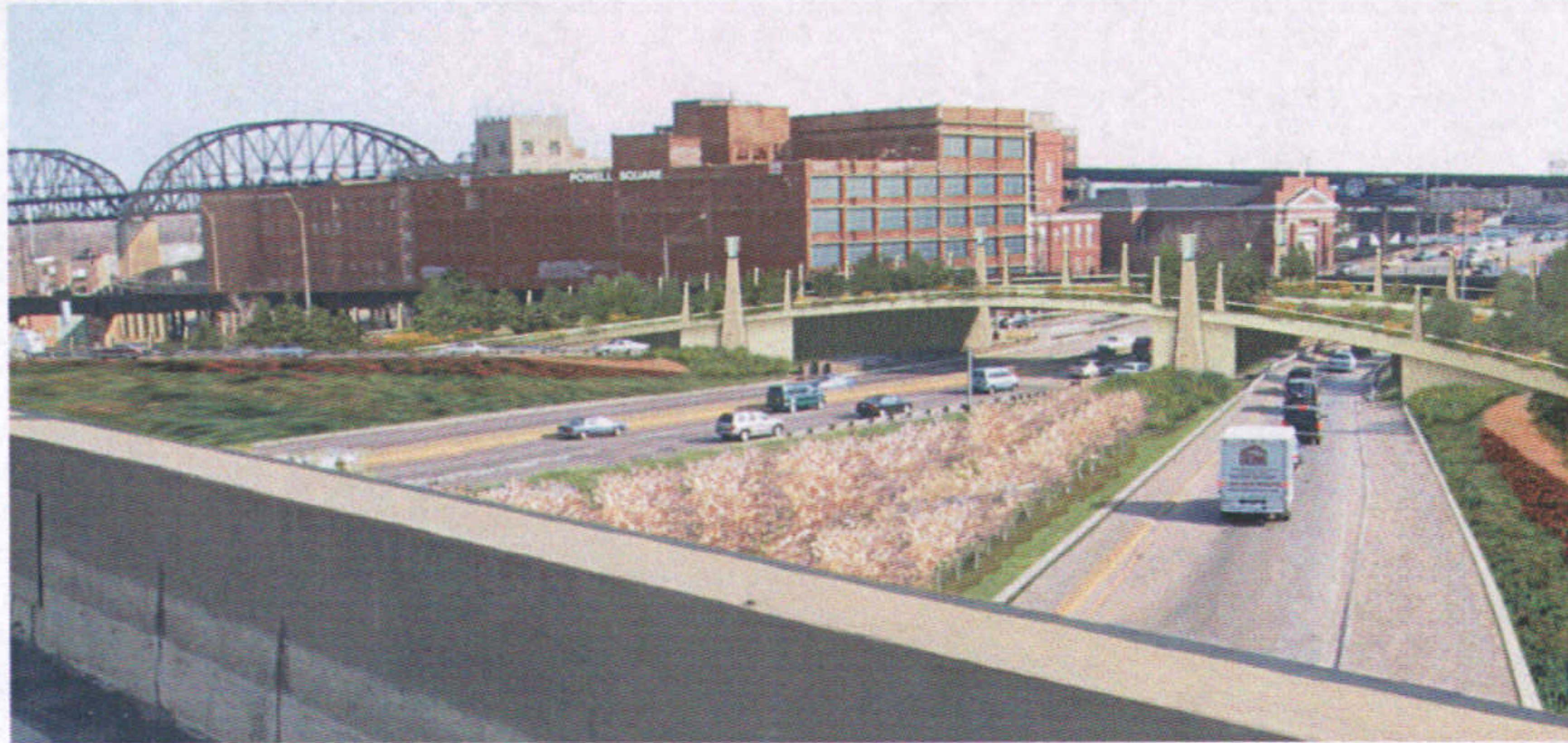
I-55 pedestrian bridge
